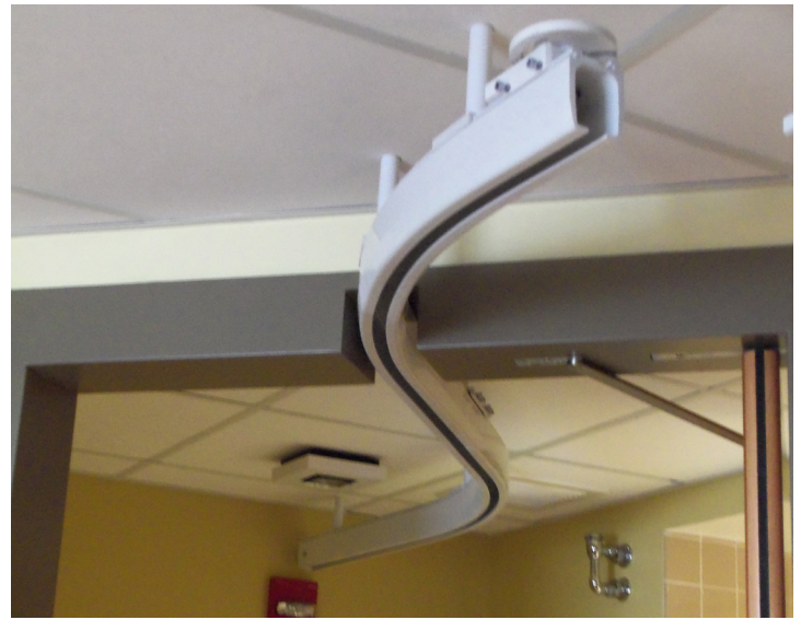
Moving gantry systems are joined to stationary tracks using the gate. These photos show how bathroom access can be provided while using the gantry system over the bed.
