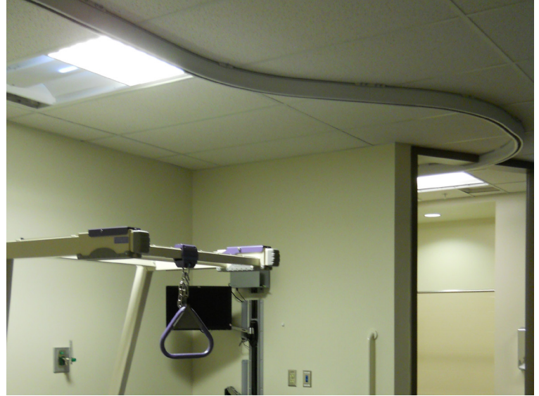
Curved track systems are designed to access other areas like bathrooms.
