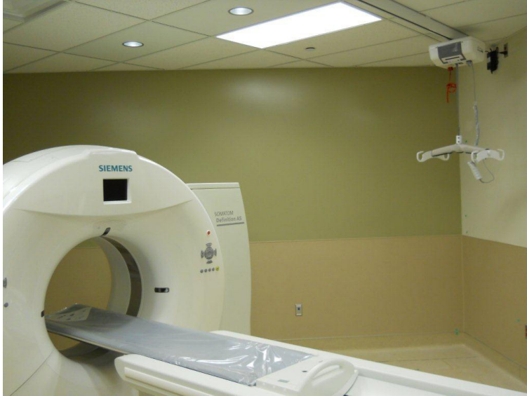
The single rail system is a popular solution for transfers in CT.
