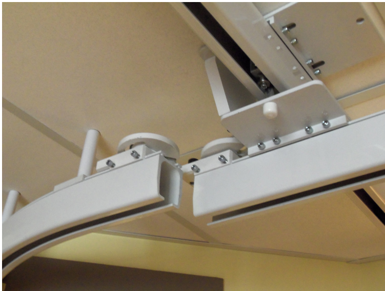
Moving gantry systems are joined to stationary tracks using the gate. These photos show how bathroom access can be provided while using the gantry system over the bed.
