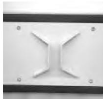
5. Safety tabs need to be checked to make sure they are installed correctly, not missing or torn.
