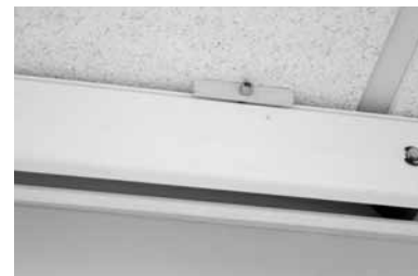
Figure 19 - Mounting Bracket
